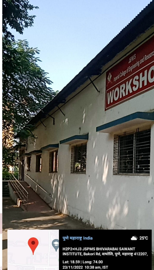
Fig 11 Ramp at central workshop of ICOER
