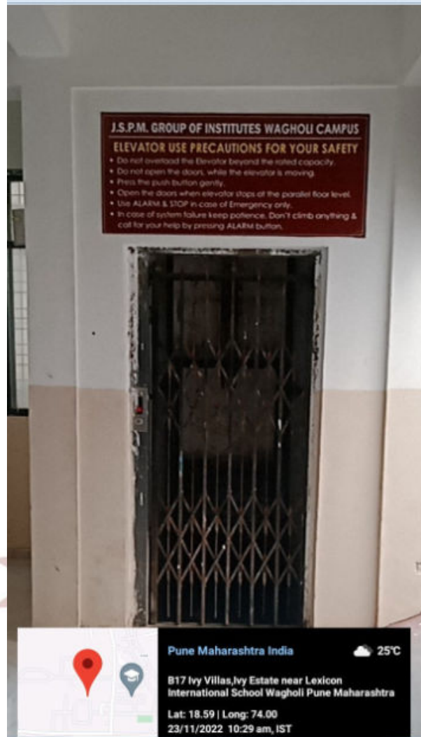
Fig. 13 Lift in building A of ICOER
