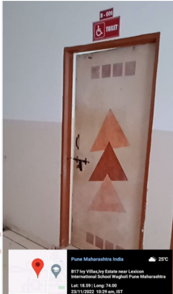
Fig. 12 Toilet for disabled of ICOER
